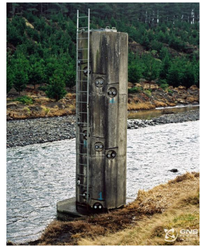
Photo 10 - Rail lahar warning system, Whangaehu River, Taupo Volcanic Zone by Lloyd Homer (Copyright: GNS Science)
